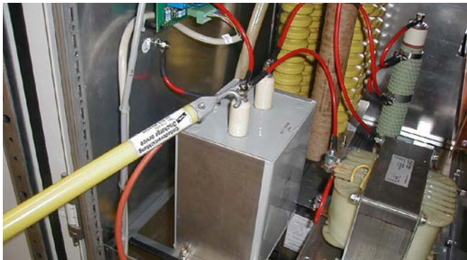
Single-pole device for discharging static charges.
