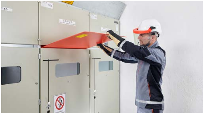
Inserting a protective shutter of type A4 into a closed system.
