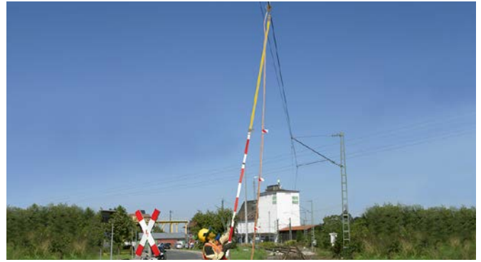
Attaching a railway earthing device.
